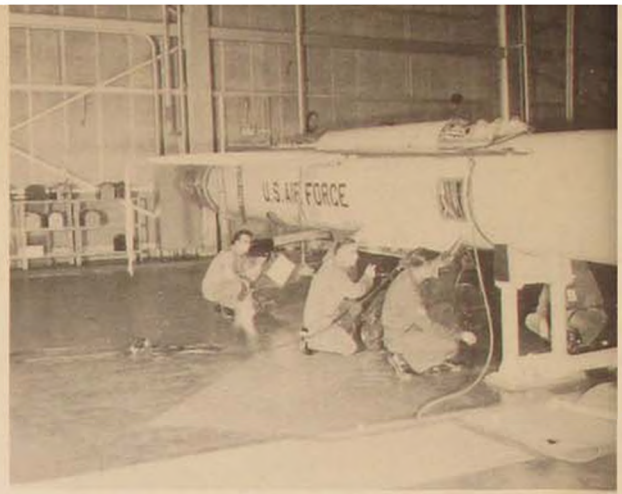
Preparing the missile forward for the installation of its two ramjet engines.
