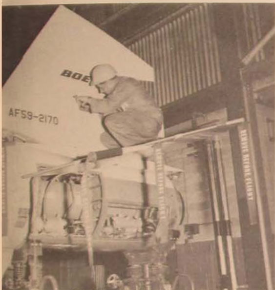
A missile squadron technician installs antenna on the vertical stabilizer.
