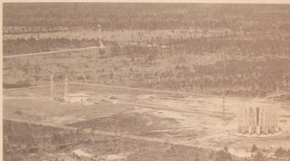
The Bomarc weapon system ground-to-air transmitters (GAT) at Hurlburt Field, Eglin Air Force Base, Florida. At left are the two omnidirectional tower antennas of the IM-99A Bomarc GAT and at right the directional horns of the IM-99B GAT antenna.
