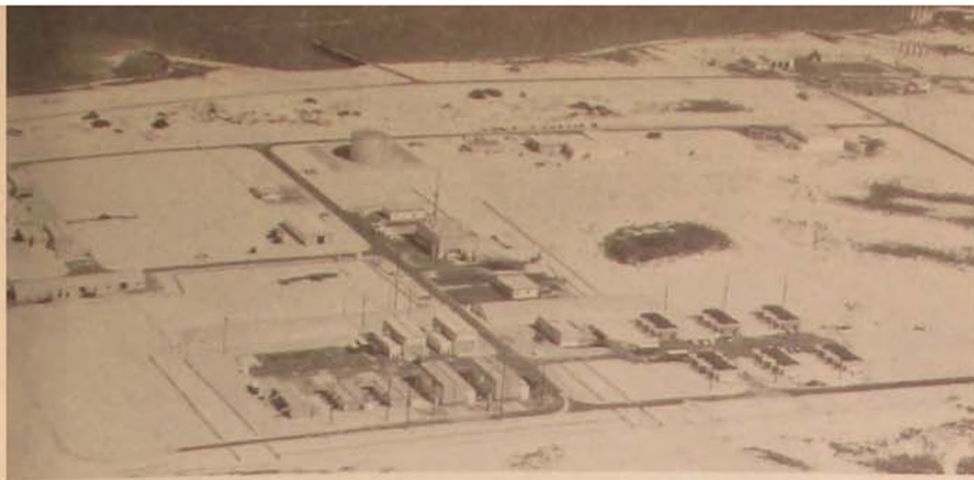
The combined Bomarc IM-99A and IM-99B testing facilities, Santa Rosa Island, Florida. In the foreground "A" shelter launchers are on the left and "B" shelters on the right.
