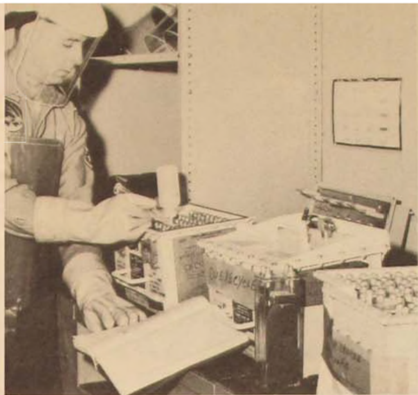
Servicing a 52-volt servobattery, which powers Bomarc hydraulic system. Protective equipment prevents splatter burns.
